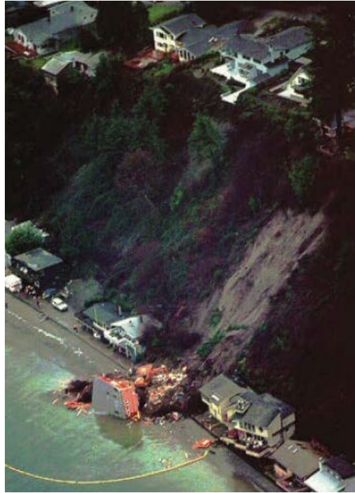
Figure 7.6 Rolling Bay, Bainbridge Island 1997 2 Landslide Type: Debris Flow
